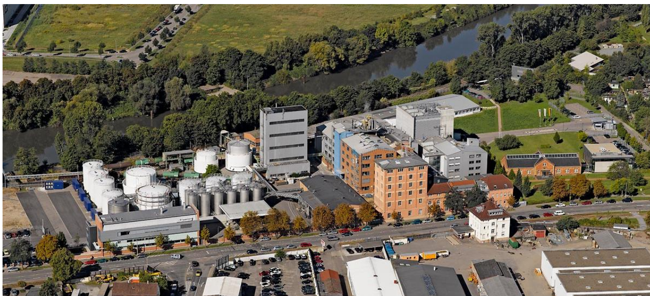
figure 1: Headquarter of Brüggemann in Heilbronn at the Neckar River
